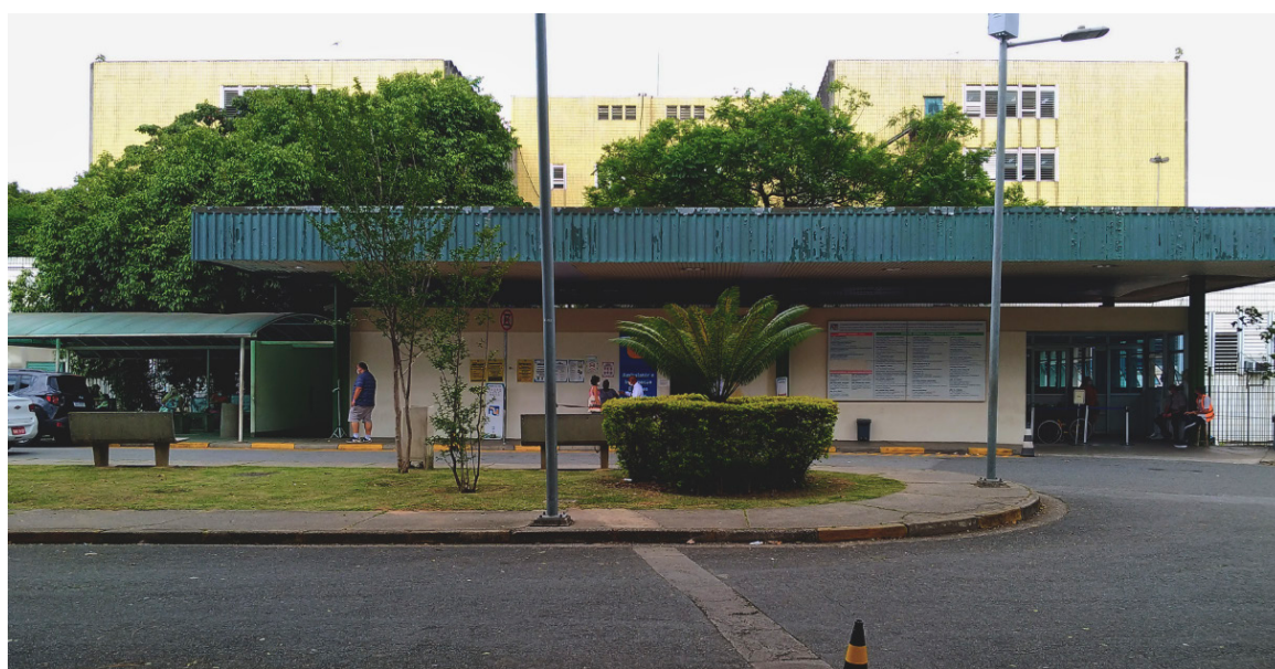
Illustration 4 . Access to the administrative floor and to the public. Source: Authors.
