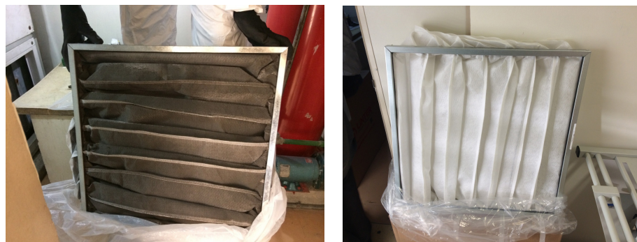
Pictures 2 and 3 – Replacing F7 saturated bag filters, August 2017 Credit: Personal collection.
