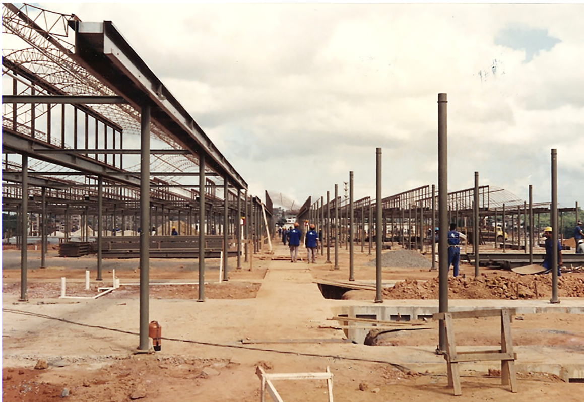
Illustration 13. Sarah/BA - assembly of double longitudinal beams and transversal tie beams. Source. Photograph Haroldo Pinheiro. Author's personal archives.
