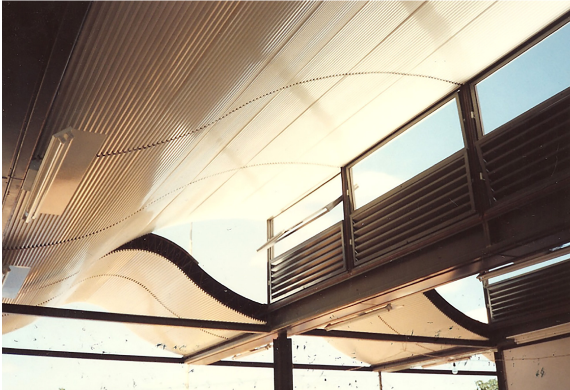
Illustration 15. Sarah/BA - double beams with attached light fixtures, tie beams and roof being assembled: foreground with shed; background, without shed (for balconies and air-conditioned rooms). Source. Photograph Haroldo Pinheiro. Author's personal archives.
