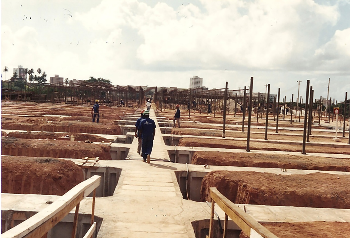
Illustration 11. Sarah/BA – gallery network with dentils to assemble tubular pillars.
