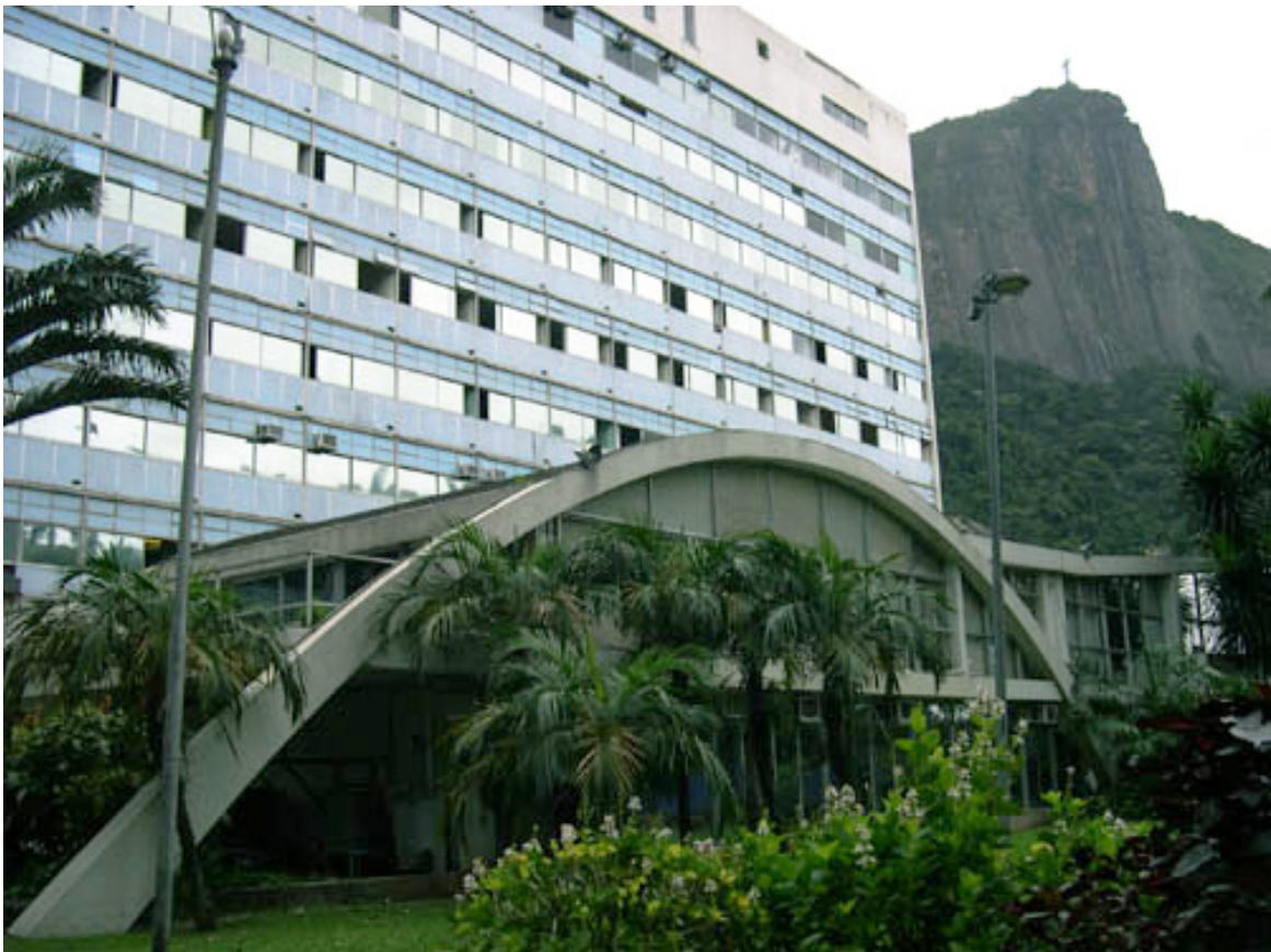
Picture 5. East façade of Hospital da Lagoa. Source: Rio de Janeiro - NEMS, 2012.
