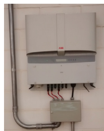
Illustration 13: Installation of a string photovoltaic inverter Source: Solstício Energia 2016
