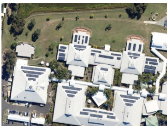
Illustration 19: A system connected to a 266kW grid with 38 string inverters in Pialba, Australia, which has been designed considering the photovoltaic system from its inception and has been optimized to receive the grid-tie Source: ABB, 2013
