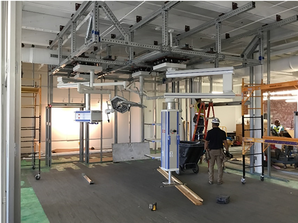
Figure 8. Overhead boom and light structure
