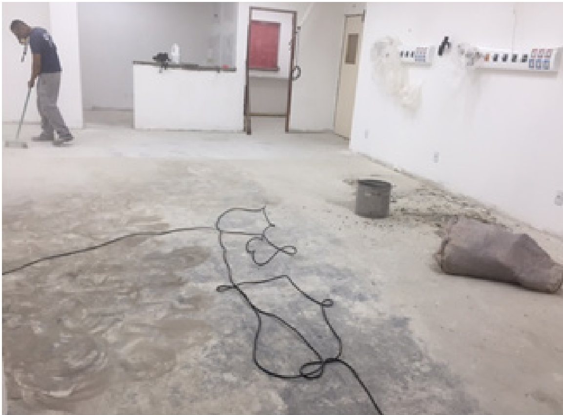
Illustration 3. Removal of dirt from the floor for the application of the vinyl blanket. Source: Own authorship (2017).
