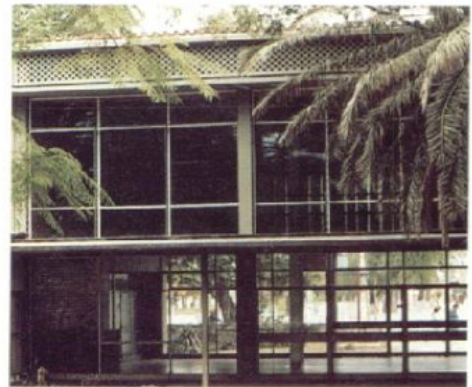
VISTA EXTERIOR HALL
