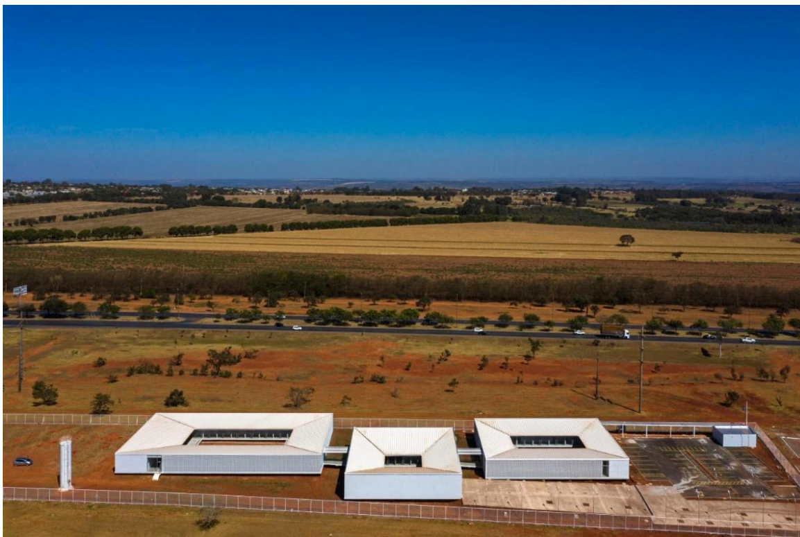
Illustration 4. Aerial view of UBS-5, from its left elevation (northeast) Source: Saboia+Ruiz Architects
